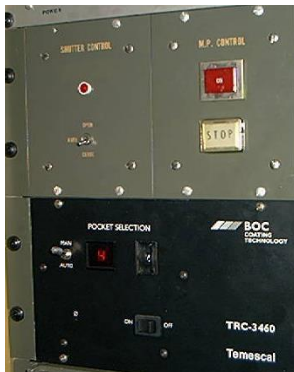
Figure 4: Shutter Control (Top Left), Mechanical pump Control (Top Right), and Pocket Selector (Bottom).
